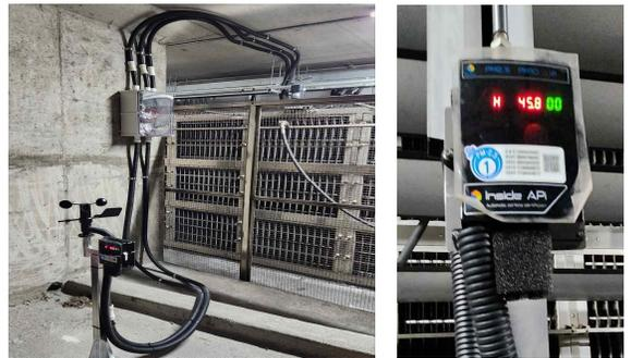
Fig. 4 Anemometer(left), Fine dust sensor(right)
