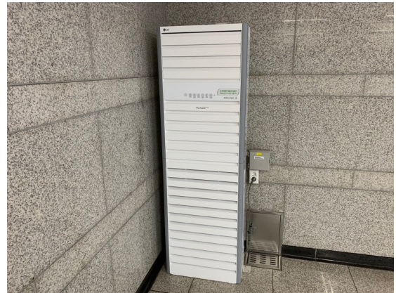
Fig. 2 Installation of Air Purifier in DJET
