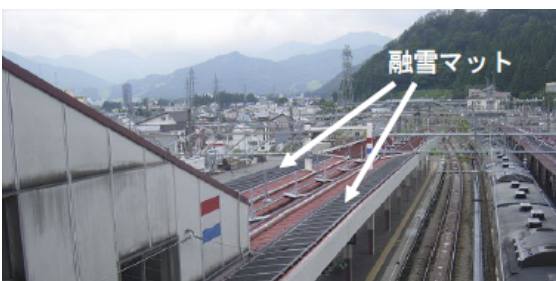
Fig. 2 Roof Snow Melting Control System
