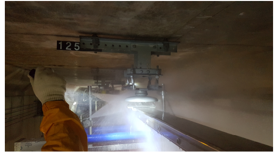
Fig. 2 Insulator cleaning with spray nozzle
