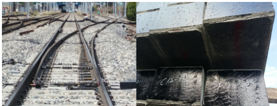
Fig 1. Sample construction of USP Turnout
