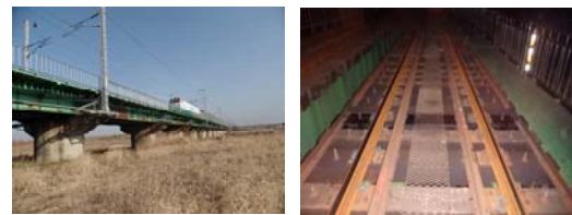
Fig. 1 Steel Plate Girder
