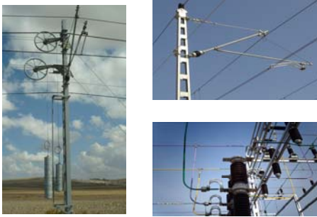
Fig. 2 Tensioning device and Moveable Bracket, Substation insulator in Spain[3]
