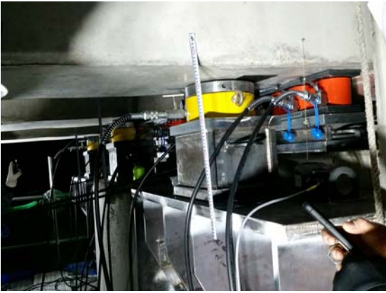
Fig. 2 Lifting process of beam structures
