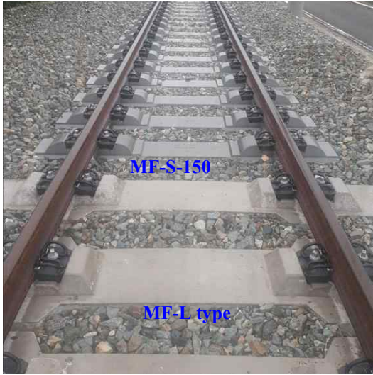
Fig. 1 Field installation of wide sleepers in ballasted track
