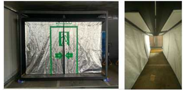
Fig. 3 In the ceiling type deployable safe pathway
