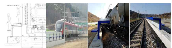
Fig. 1 Low height soundproofing apparatus site construction section and installed photos.
