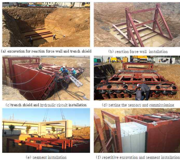
Fig. 2 Construction Sequence of Trench Shield
