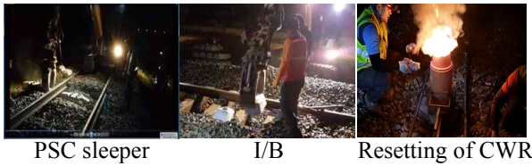
Fig. 2 Installation procedure of new track structure
