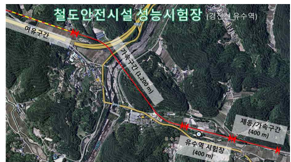
Fig. 1 The performance test site
