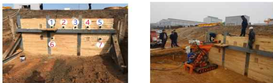
(a) Construction Step (b) Construction View Fig. 4. SEM-Pile Construction
