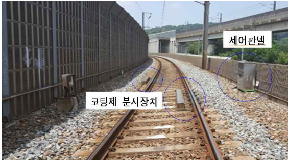
Fig. 2 Rail Coating System installation site
