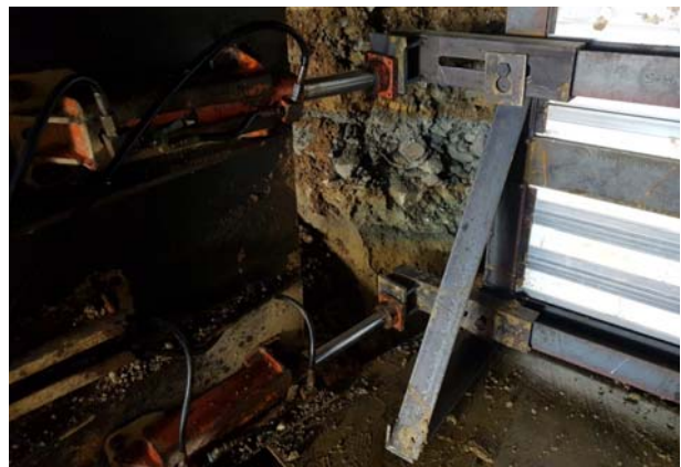
(b) Hydraulic jack installation
