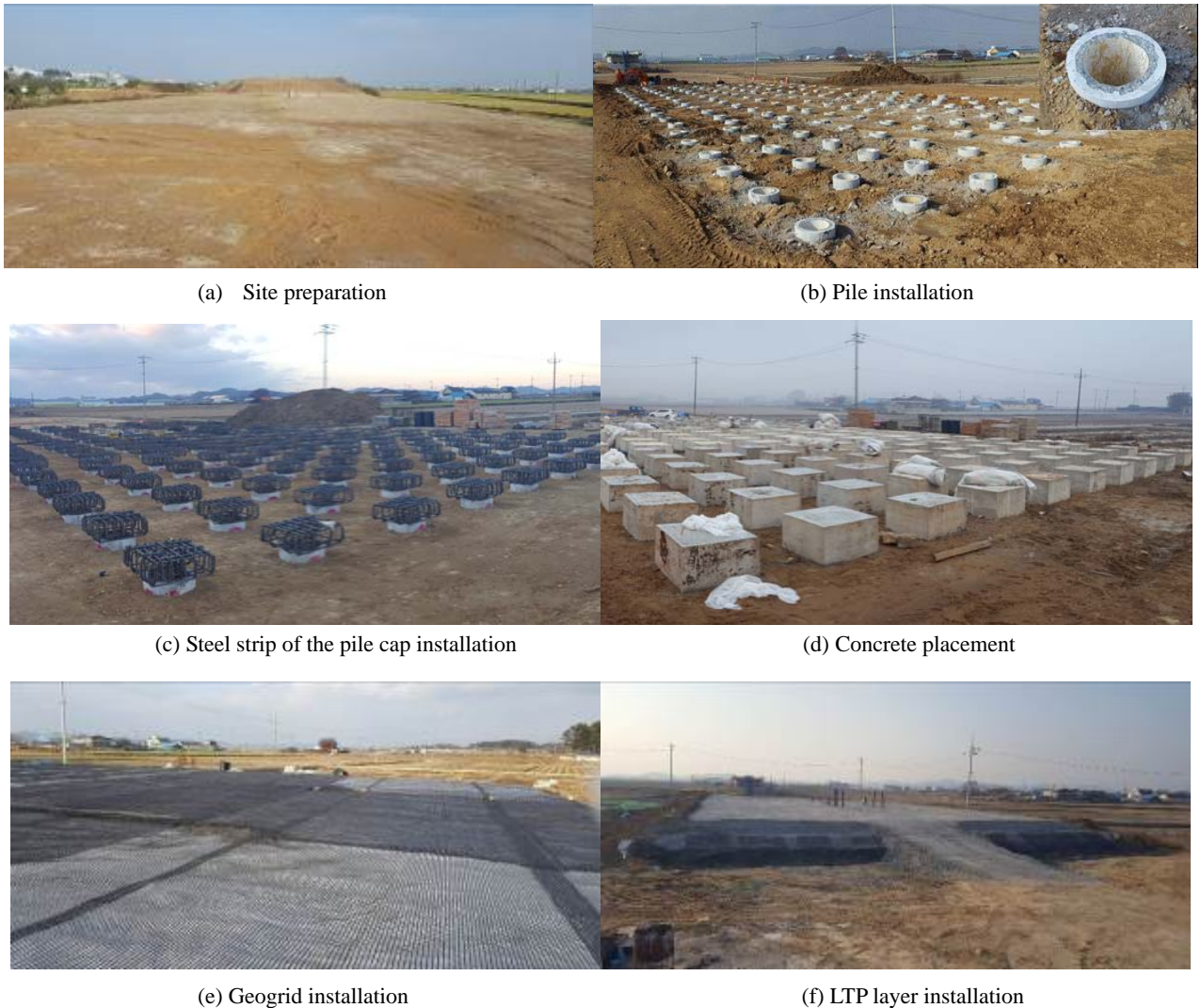
Fig. 4 Test-Bed construction sequence
