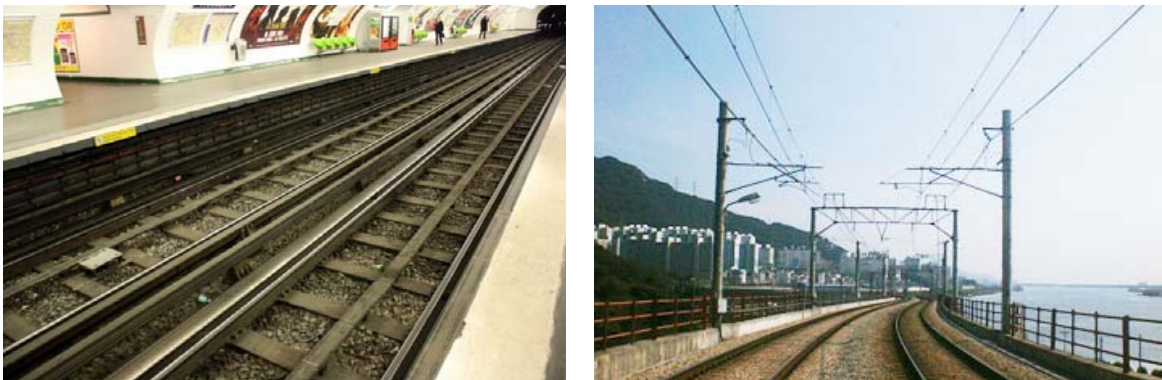
Fig. 1 Third-Rail and Overhead Catenary feeding Method
