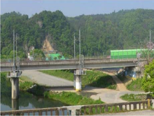
Fig. 1 Selected bridge (Sumjingang 1 bridge)
