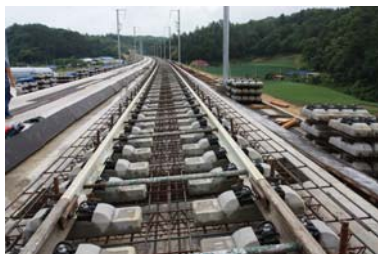
Fig. 3 Setting the track before pouring concrete
