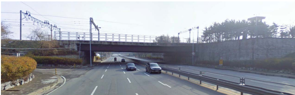
Fig.2 View site of line No.8
