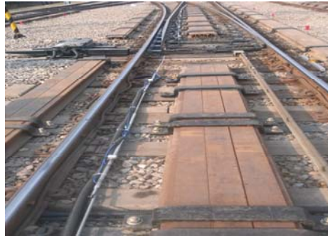
Fig.3 View of measurement
