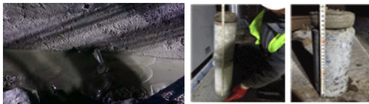
Fig. 7 Check the Charge of Cement Mortar
