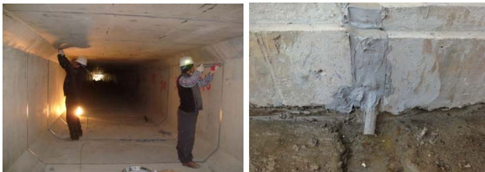
(a) Water-proof work
