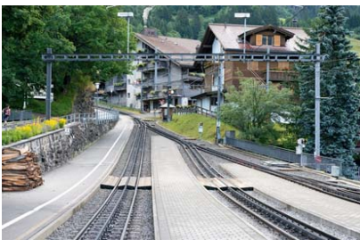
(a) Mountain railway track Structure
