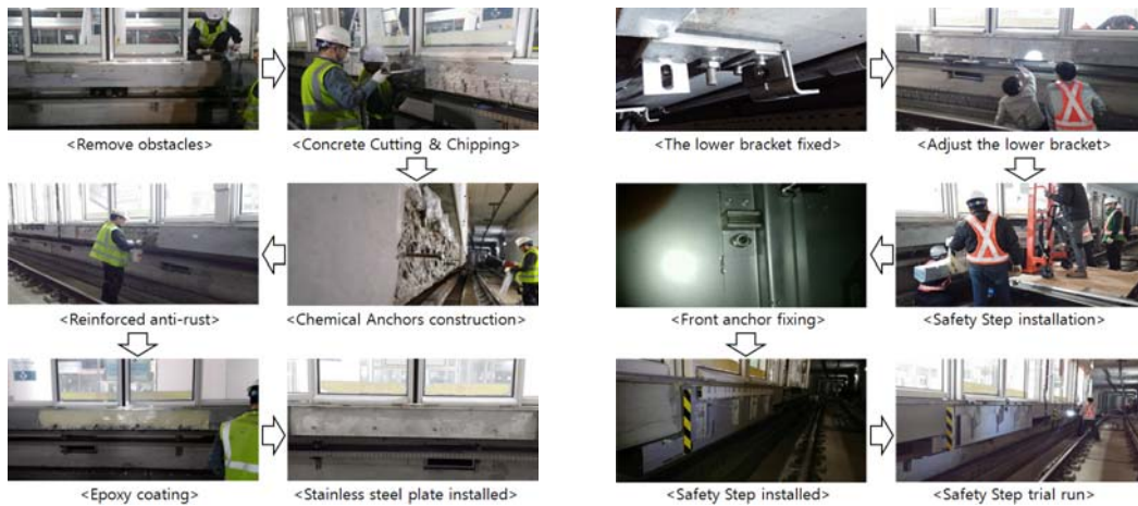
(a) Platform Safety Step Construction Procedure
