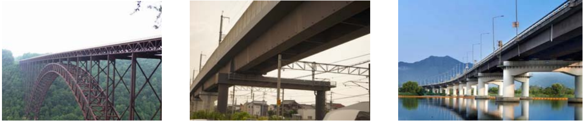
(a) New River George Bridge (U.S.A.) (b) Matsubara Railway Bridge (Japan) (c) Yang-su Bridge (Korea)
