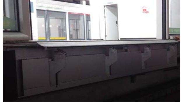
Fig 7. Installation of the safety scaffolding
