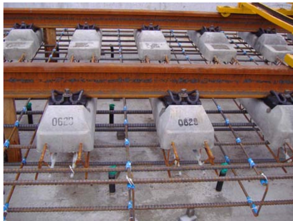
Fig. 8 Insulation of reinforcing bars[3]
