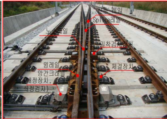
Fig.2 Movable nose crossing (concrete track)
