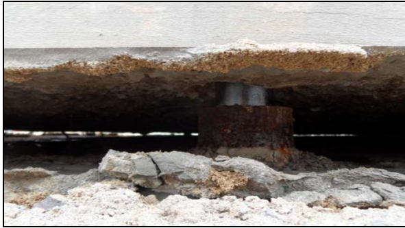
Figure 2. Rail Jack-up Test
