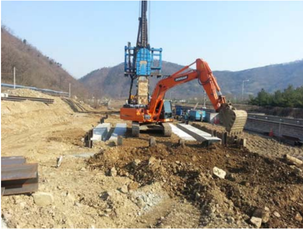
Fig. 5 construction of cab beam
