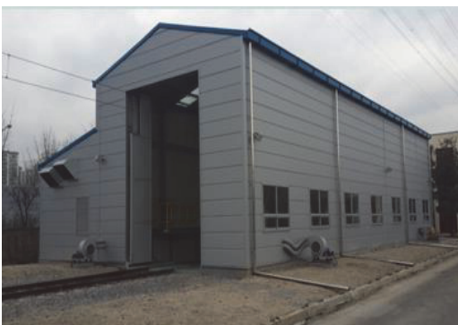
Fig. 5 The exterior of the lower washing equipment
