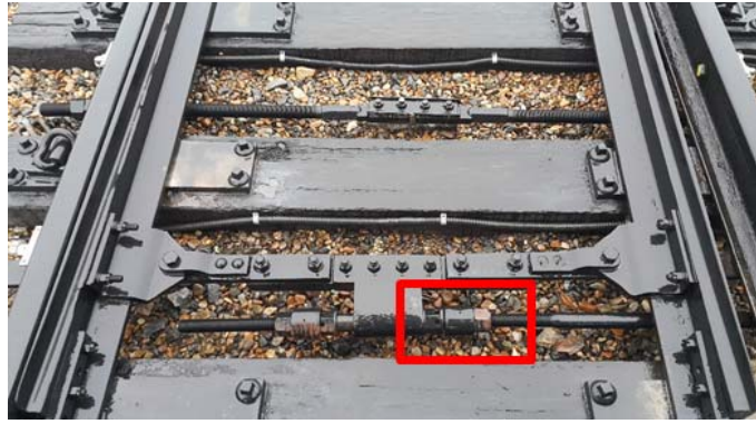
Fig. 3 Photo of Drive rod with slacked nut
