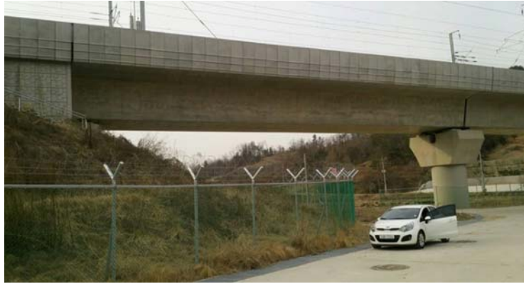
Fig. 1 View of the bridge
