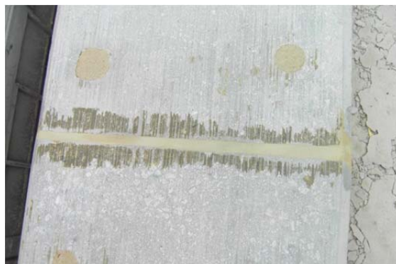
Fig. 8 Application method the filler between the panel and the panel
