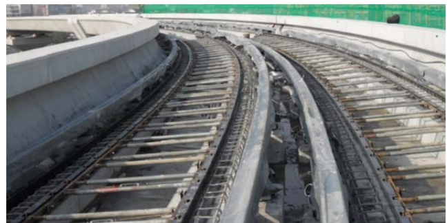
Fig. 6 Install formwork of Filling
