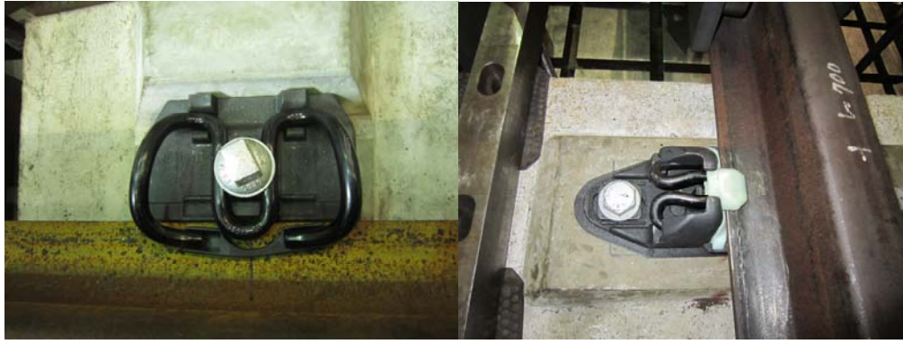
(a) A type rail fastening system
