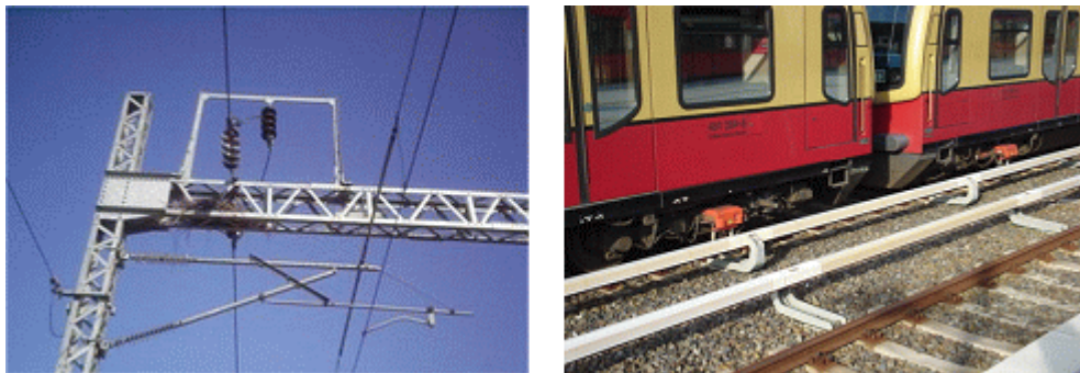
Fig. 1 Overhead Catenary and Third Rail Feeding Method
