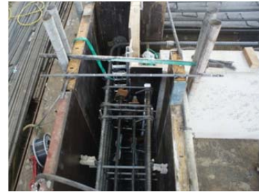
(c) WS#3(Coupler+T bolt)
