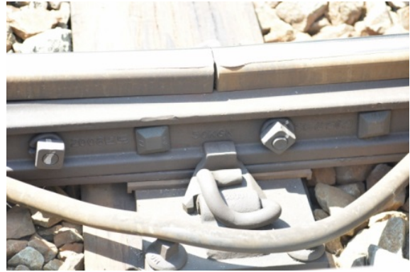
Fig.3 Close-up picture of the Rail joint
