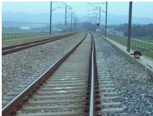
Fig. 3 Alignment irregularity symptoms
