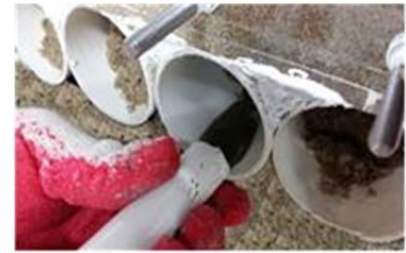
(c) Remove the Soil inside the Steel Pipe, Concreting
