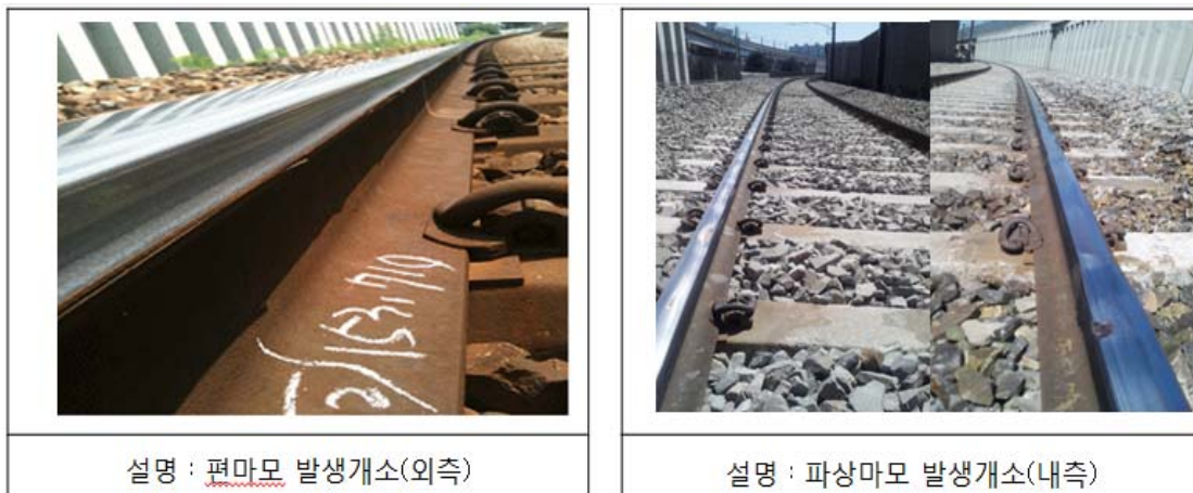
Fig. 2 DaeJeon-buk connection line T2 track
