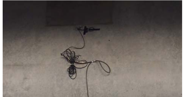
(b) The installed accelerometer
