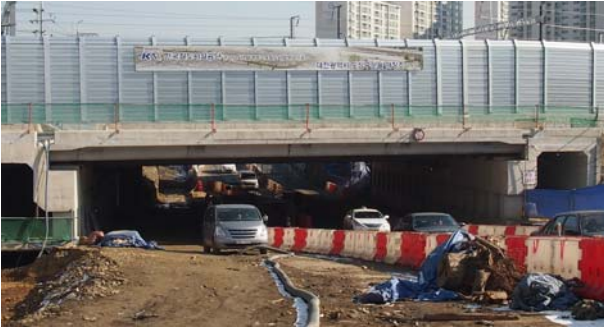
(a) View of measured bridge
