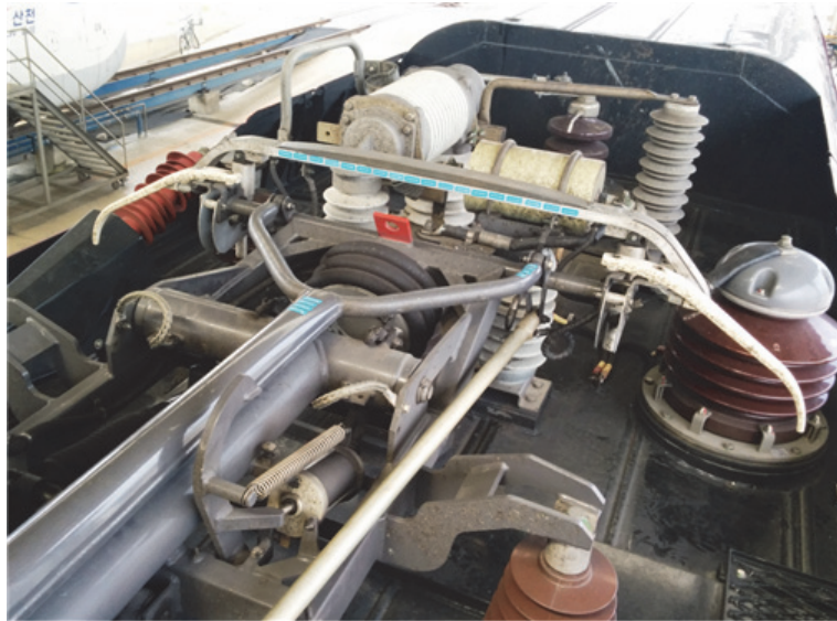
Fig. 2 Thermo tape application on pantograph
