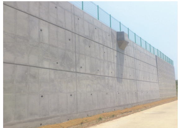
Fig. 2 View after construction
