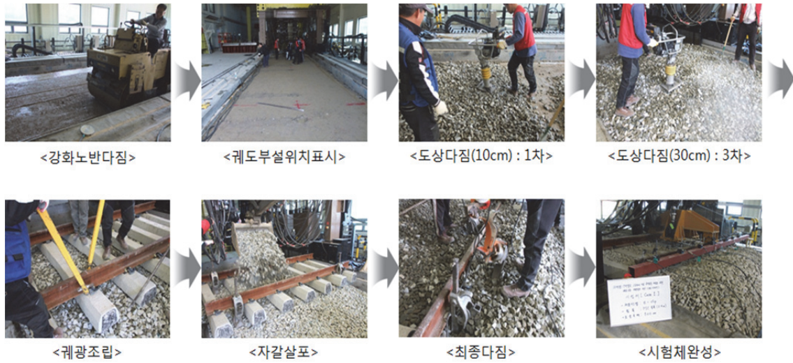
Fig. 4 Construction processes of full-scale specimens
